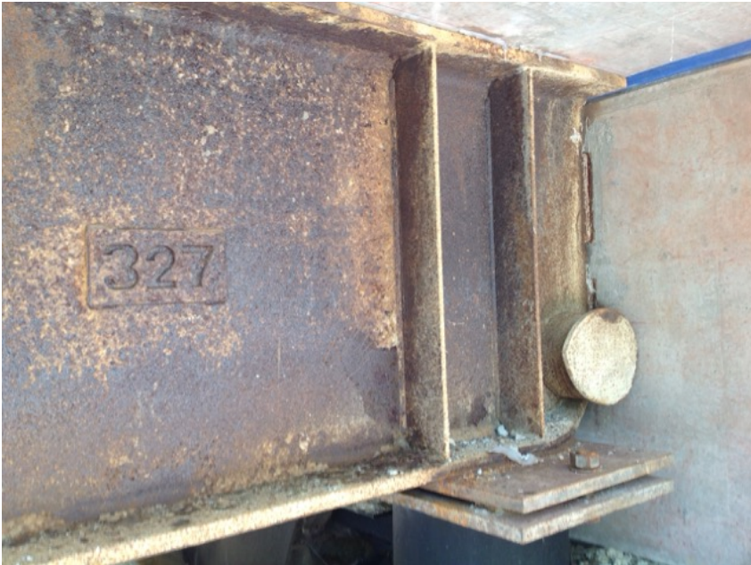
recycled steel girders
