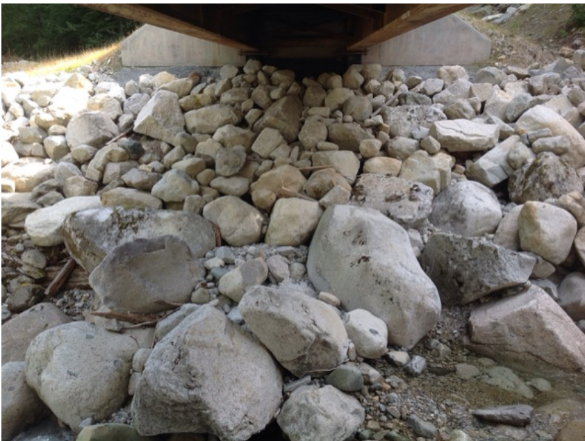
Right Bank Abutment when facing downstream
