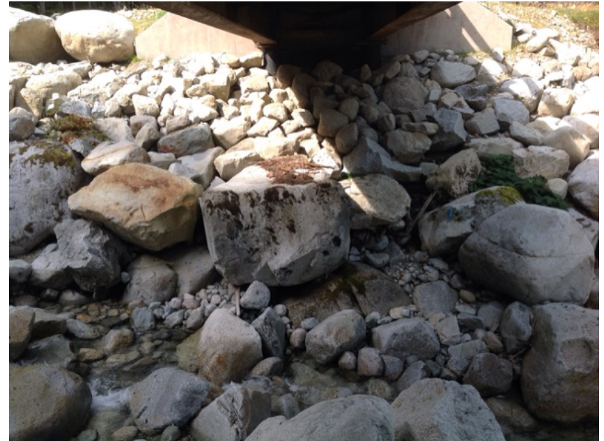
Left Bank Abutment when facing downstream
